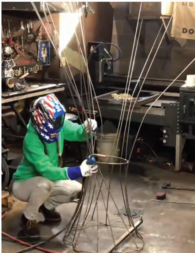
Fig. 3 — Barbie the Welder uses a ¼-in. round bar to build the frame of the statue's body.
